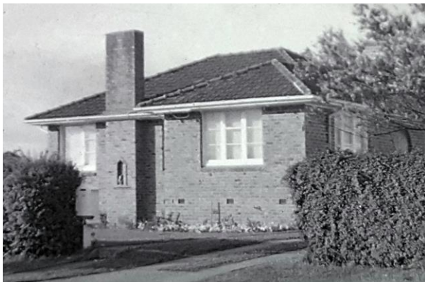
14 Burns Ave, Takapuna
